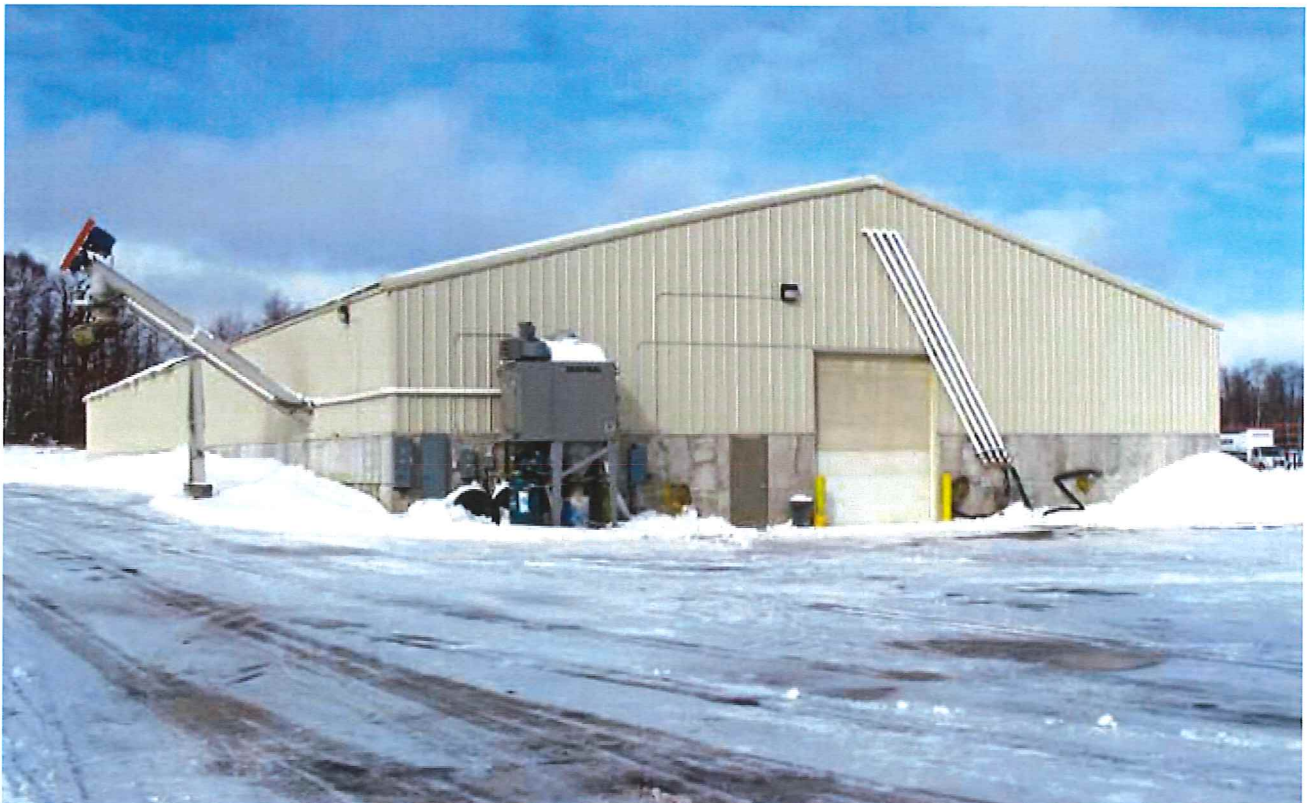
Photo 1: National Minerals Corporation's terminal in Cohasset, MN, allows storage of ash produced during winter months for use in the summer construction season
